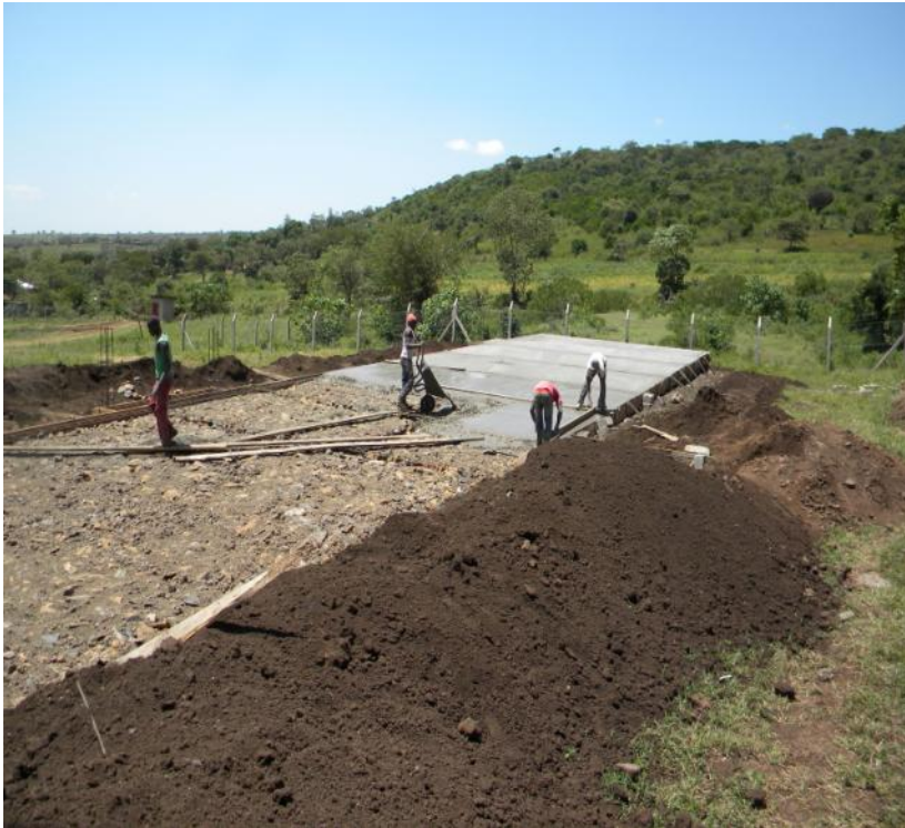
Foundation being poured for Tanzania Christian academy student housing
