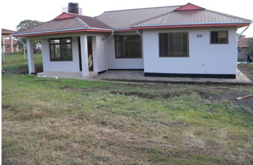
Newly completed headmaster's house at Tanzania Christian Academy
